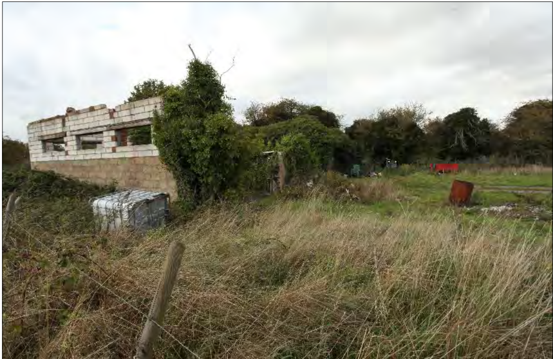
Plate 44: Bowaters Farm: View of the southern range of Cold War buildings, facing southwest
