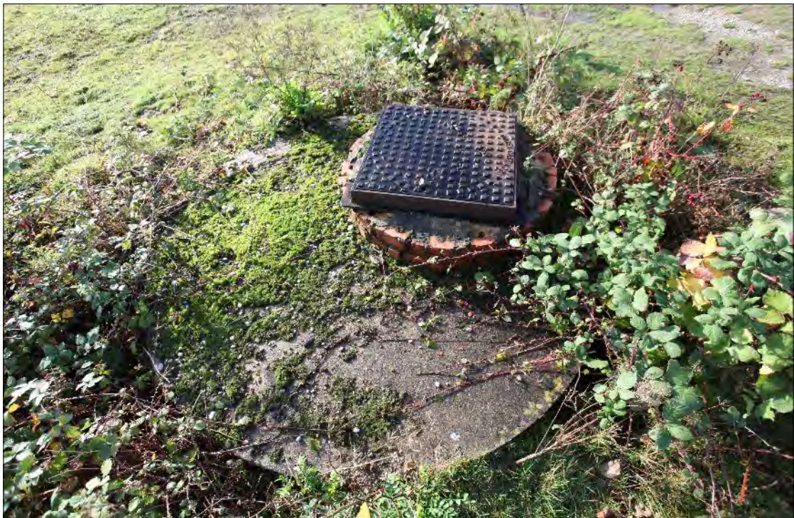
Plate 20: Orsett: modern manhole on earlier concrete structure?
